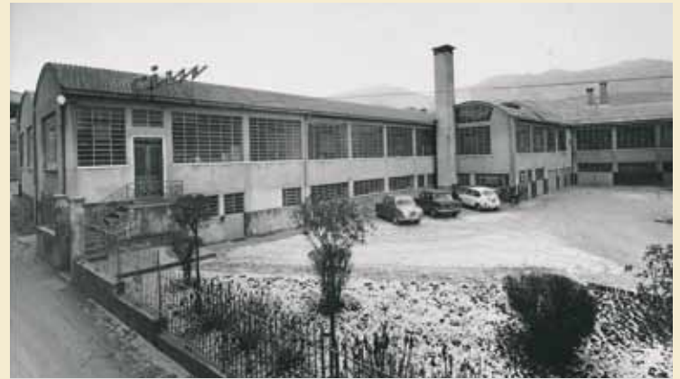
Primo stabilimento Cimberio 1957 Cimberio's first manufacturing facility in 1957
