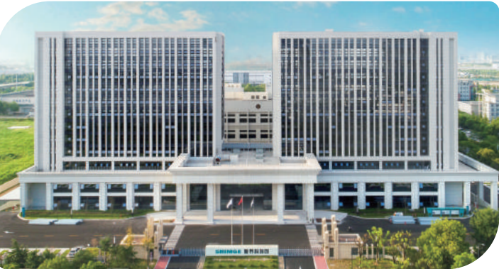
Shimge's production base in HangZhou, Zhejiang Province
