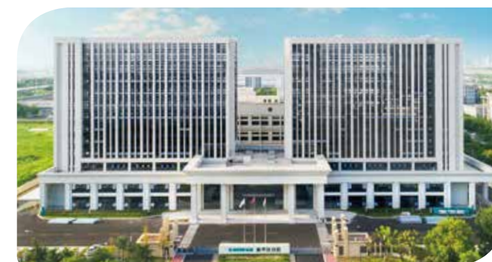
Shimge's production base in HangZhou, Zhejiang Province
